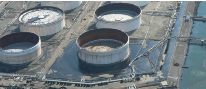
Leakage of hazardous materials from an outside storage tank - in the Great East Japan Earthquake (courtesy of Sendai City Fire Bureau) 屋外タンク貯蔵所からの危険物流出/東日本大震災 (仙台市消防局提供)
