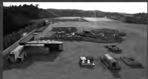
USAR Training Facility HYOGO
