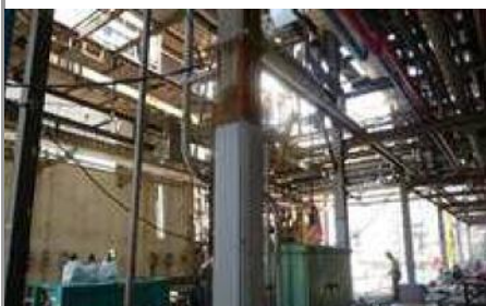
柱に 12~19mm 鋼板を溶接補強
