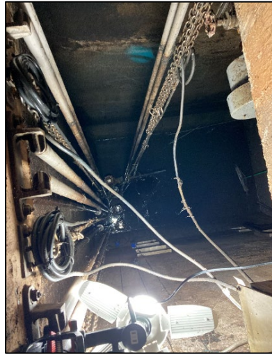
① [西側汚泥槽 (要救助者転落槽)]
